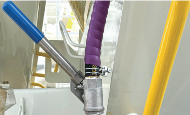
4.Spring loaded switch for water charging.
