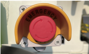
7.Emergency stop buttons: Four Emergence Stop buttons applied and covered by protections.
